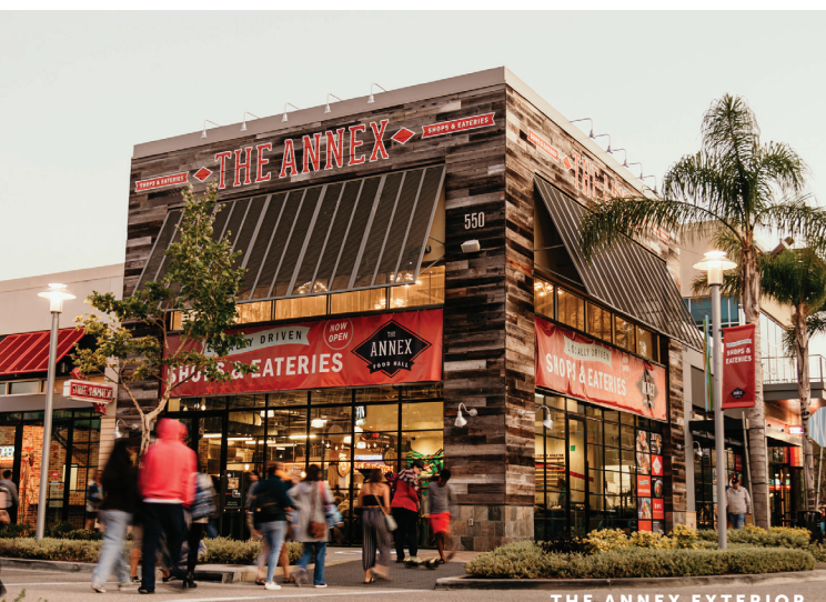
THE ANNEX EXTERIOR
